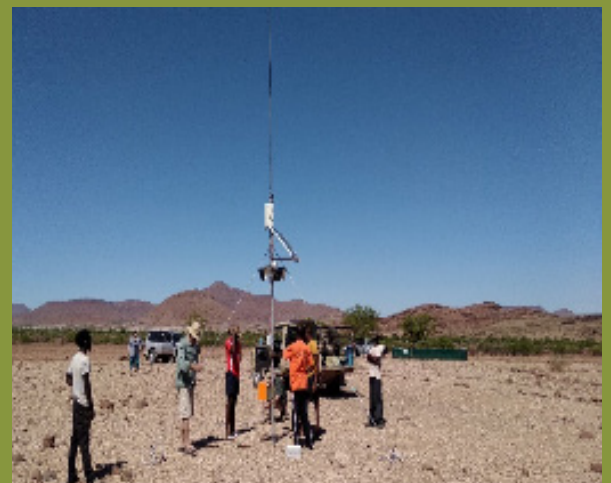
RRT erecting EW tower at Okaturua, Anabeb
